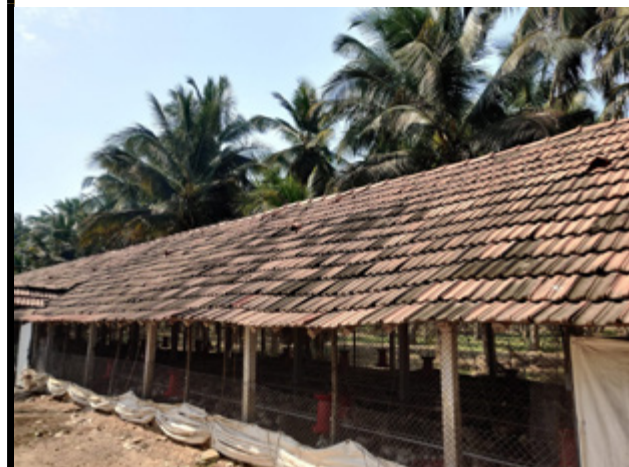
Figure 95 Example of typical open-sided housing.
