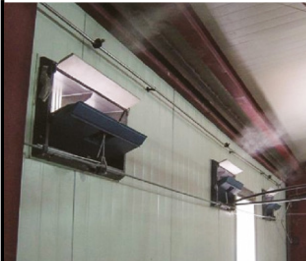
Figure 112 Example fogging system for a cross-ventilated house.
