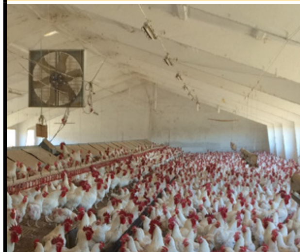
Figure 96 Circulation fans in an open-sided / naturally ventilated house.
